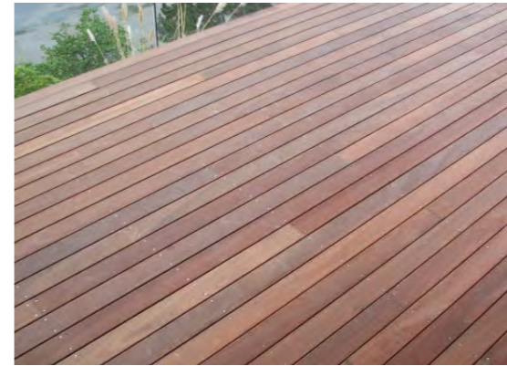
TIMBER DECKING ROOFTOP
