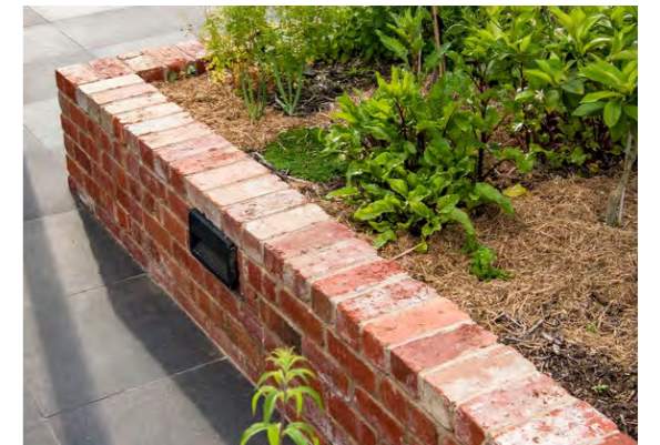
RECYCLED BRICK PLANTER
